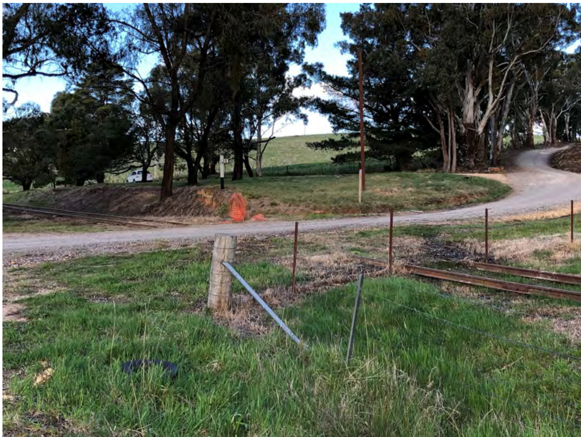
Figure 22 Level crossing reinstated over existing track at Black Bullock Road
