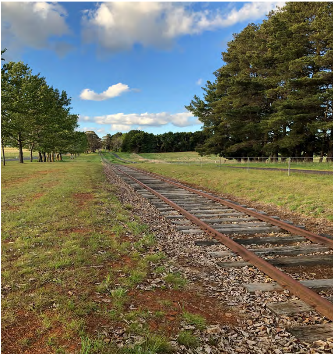
Figure 20 Existing Oberon to Tarana railway near Oberon
